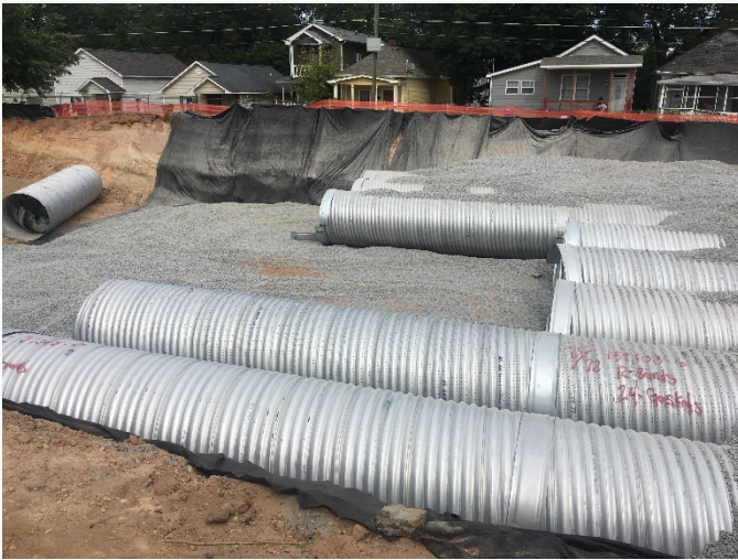
Installation and backfill of UDS
