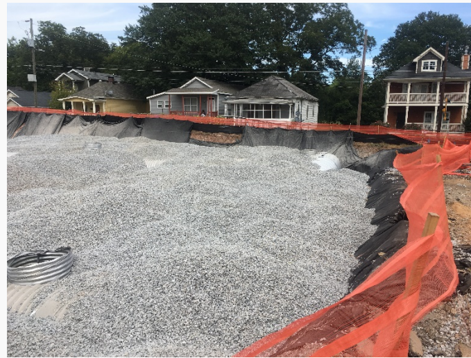
Installation and backfill of UDS
